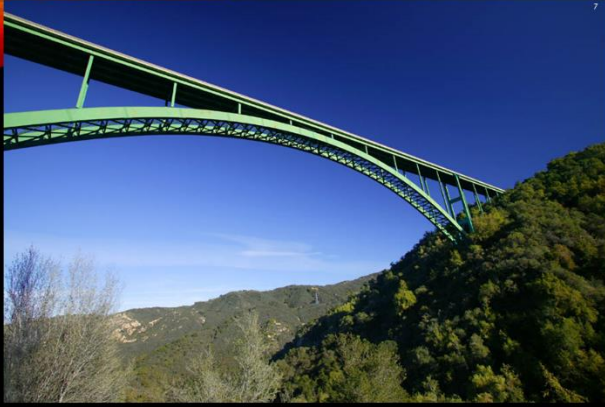
Cold Spring Arch Bridge, Santa Barbara, CA
