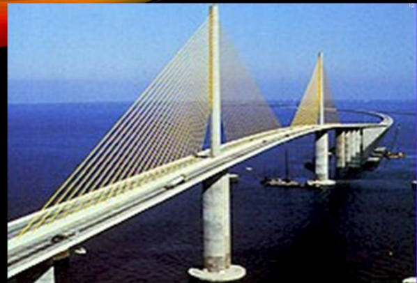
Sunshine Skyway Bridge, Tampa, FL
